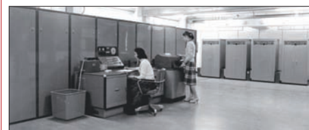
The Ferranti Mercury in building 2 in 1958.
